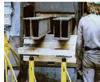
Replacing adjustment rolls under a fly-over with RR cylinders, for controlled lifting an lowering.
